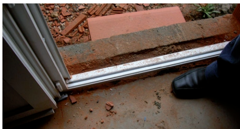
Photo: © GIE SOCATAT
