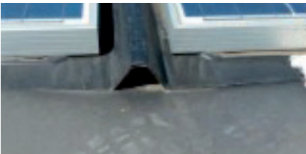
Photo : © SARETEC - Pierre LAMORIL
