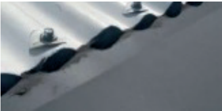
Photo : © SARETEC - Pierre LAMORIL
