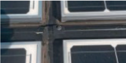
Photo : © SARETEC - Pierre LAMORIL
