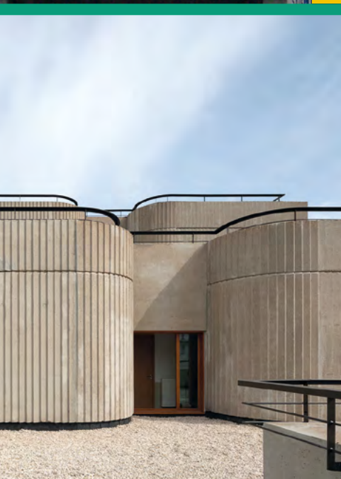
Photo © Pierre L'Excellent - Canal Architecture
