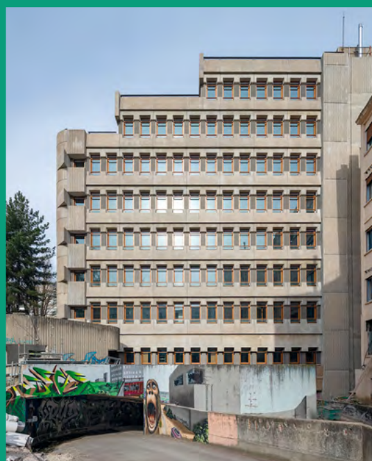
4 Photo © Pierre L'Excellent - Canal Architecture
