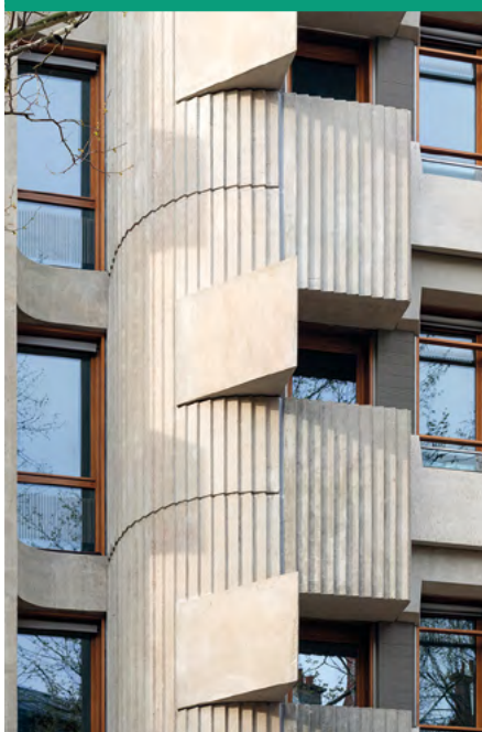
3 Photo © Pierre L'Excellent - Canal Architecture
