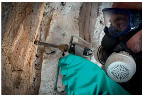
Photo © Maïndron Structures SAS
